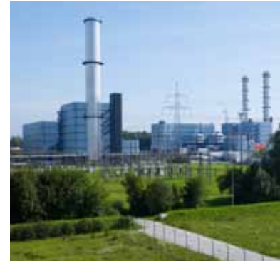
High operational flexibility due to world class fast cold start and hot restart capability
