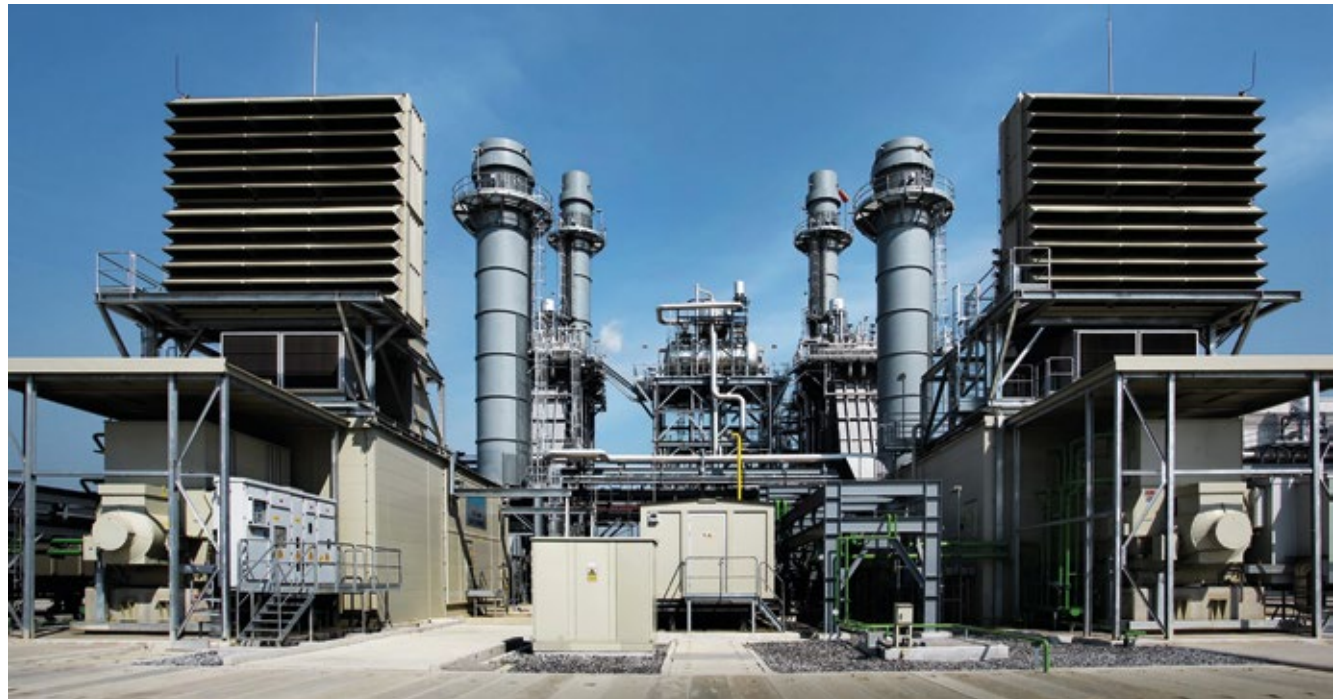
SGT-800 packages at the Amata B.Grimm Power Plant, Amata Nakorn, Chonburi, Thailand
